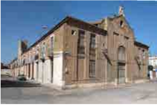
Fig. 3 - Lonja of Pescadores. View of the South façade (Photo G. Muñoz).
