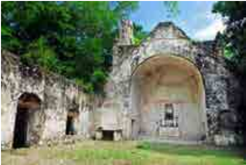
Fig. 8 - Sixteenth century Spanish chapel in Xcaret. It was built with pre-hispanic stones, and it had a maya style thatched roof. Reconstruction in Andrews and Andrews (1975).
