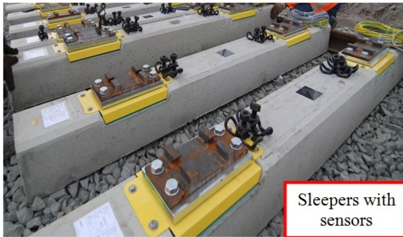
Figure 9.: Force sensitive elements placed over the sleepers
