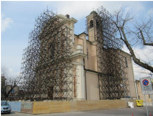
Figure 1. The church during restoration activity
