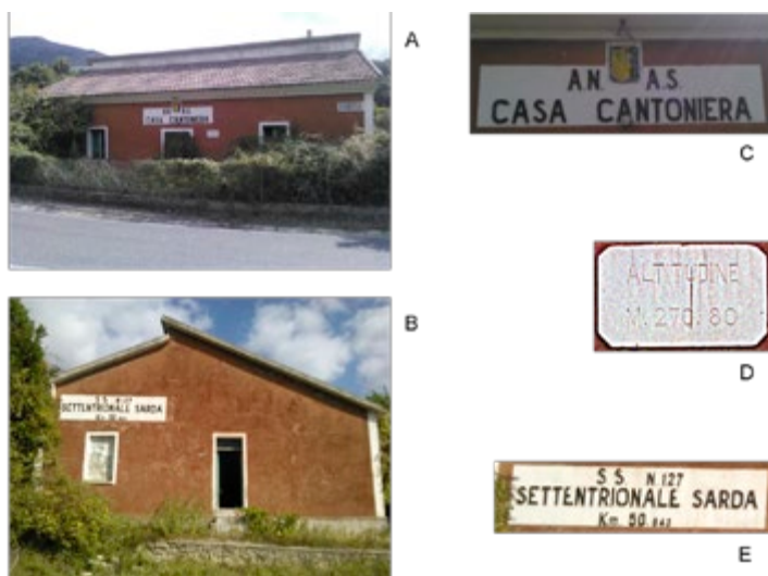
Fig. 2. An abandoned roadman's house (Northern Sardinia). A and B: two building's facades. C, D, and E: facades details. C: the typical Italian name of a roadman's house ('casa cantoniera'), decorated with the ANAS' official emblem. ANAS is the Italian acronym of 'Azienda Nazionale Autonoma delle Strade' (in English, National Autonomous Roads Corporation). D: elevation of the roadman's house above sea level (270.80 metres); letters are engraved on a plaque. E: name of the road facing the roadman's house, namely S.S. n. 127 'Settentrionale sarda': S.S. stands for 'strada statale' (in English, national road).
