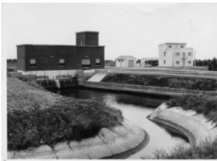
Fig. 3. Pump suction of Nova Siri _ photo year 1962 by Pietro L'Annunziata (Policoro territory).
