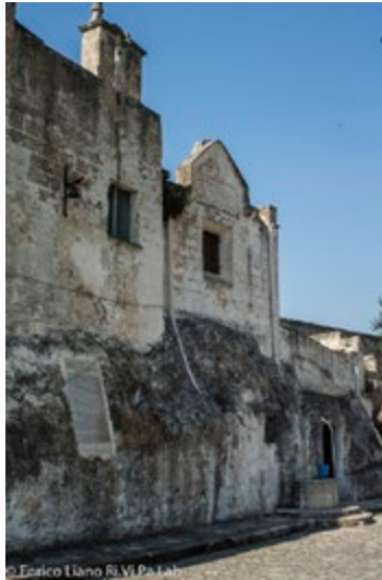
Fig. 2. Cave village near the livestock trail “tratturo” Mottola-Palagianello, Mottola (TA)
