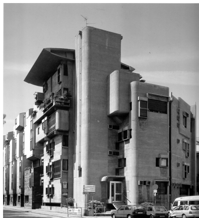
14. L. Savioli, An apartment building in Via Piagentina, Florence 1964-1966
