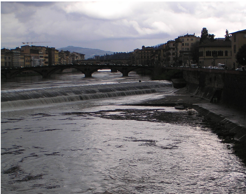
Figure 4-11: LWD and loosen material captured by eddies downstream a transversal sill, a rootwad lay down the structure for the reduced water depth (Arno River).
