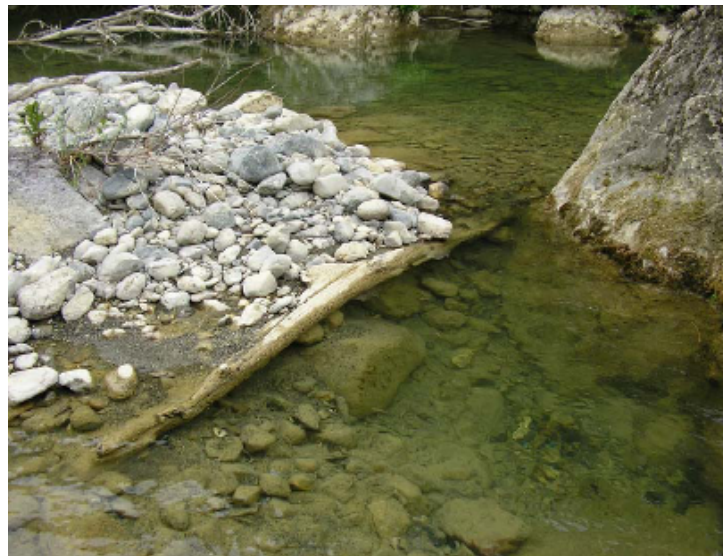
Figure 2-5: Clogged debris partially buried. (Vara River).
