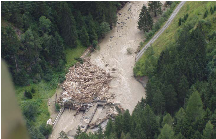
Figure 3-10: bridge obstruction an flow deviation (Passirio River, Alps).
