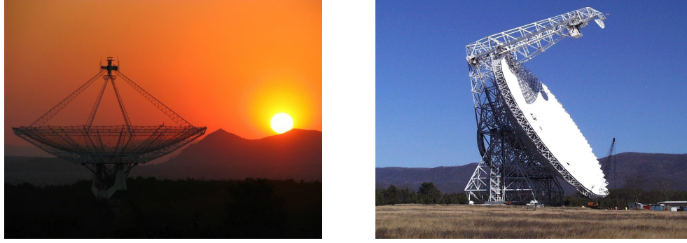
Figure 2.3: On the left: a Prime Focus 45-meters antenna of the GMRT (Giant Meterwave Radio Telescope), near Narayangaon town, India. On the right: the Green Bank Telescope (West Virginia, USA), an off-axis gregorian paraboloid of 100m diameter, the world's largest fully steerable telescope.
