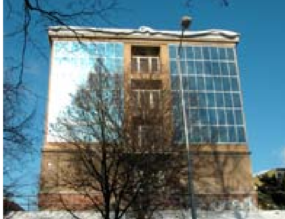
Figure 8: PV Façade with light blue solar cells manufactured by SOLARTEC for the University Liberec / CZ (Photo: SOLARTEC).
