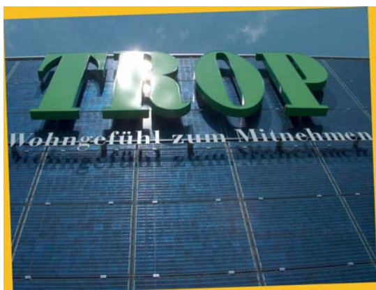
Figure 5: Façade integration of opaque PV laminates at the furniture house TROP / AT (Photo: ATB).
