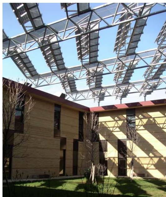
Figure 6: PV as shadowing element in the building envelope. University Florence - Sesto Fiorentino / IT (Photo: WIP).
