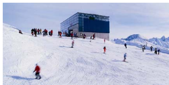
Figure 3: Façade integration of semi-transparent PV cell and PV module technology at the Kriegerhorn / AT (Photo: Sunways).
