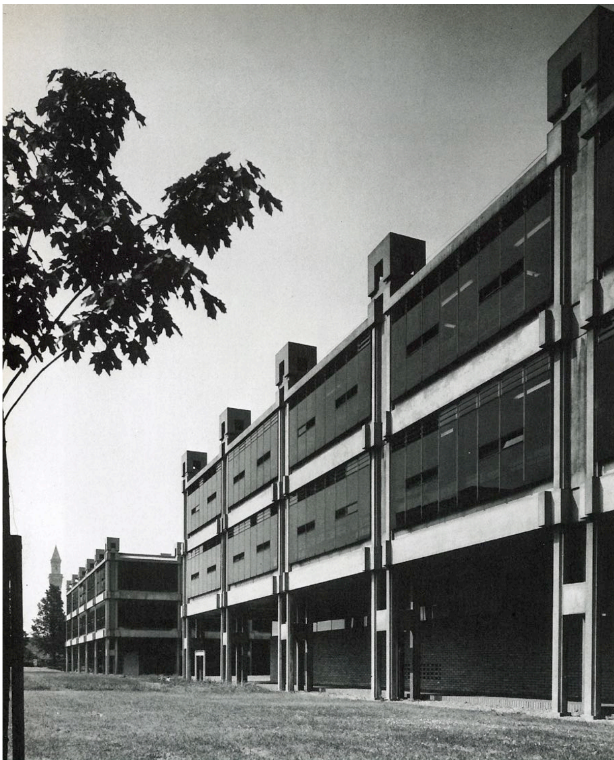
Fig. 176 - Arup Associates, Department of Mining and Metallurgy, Birmingham, (1962-66).
