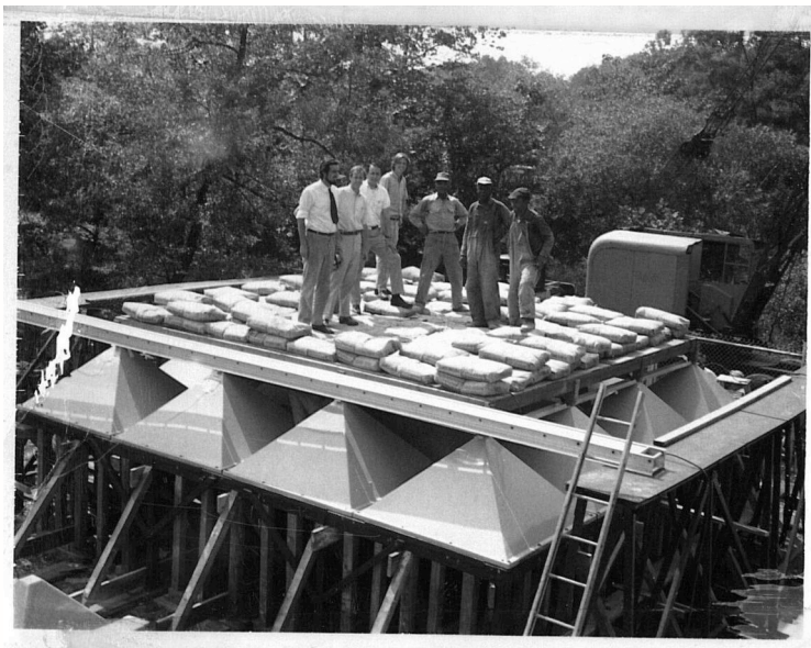
Figure 10. Renzo Piano assisted the load test of the skylight, Philadelphia, 1969. (Fondazione Renzo Piano)
