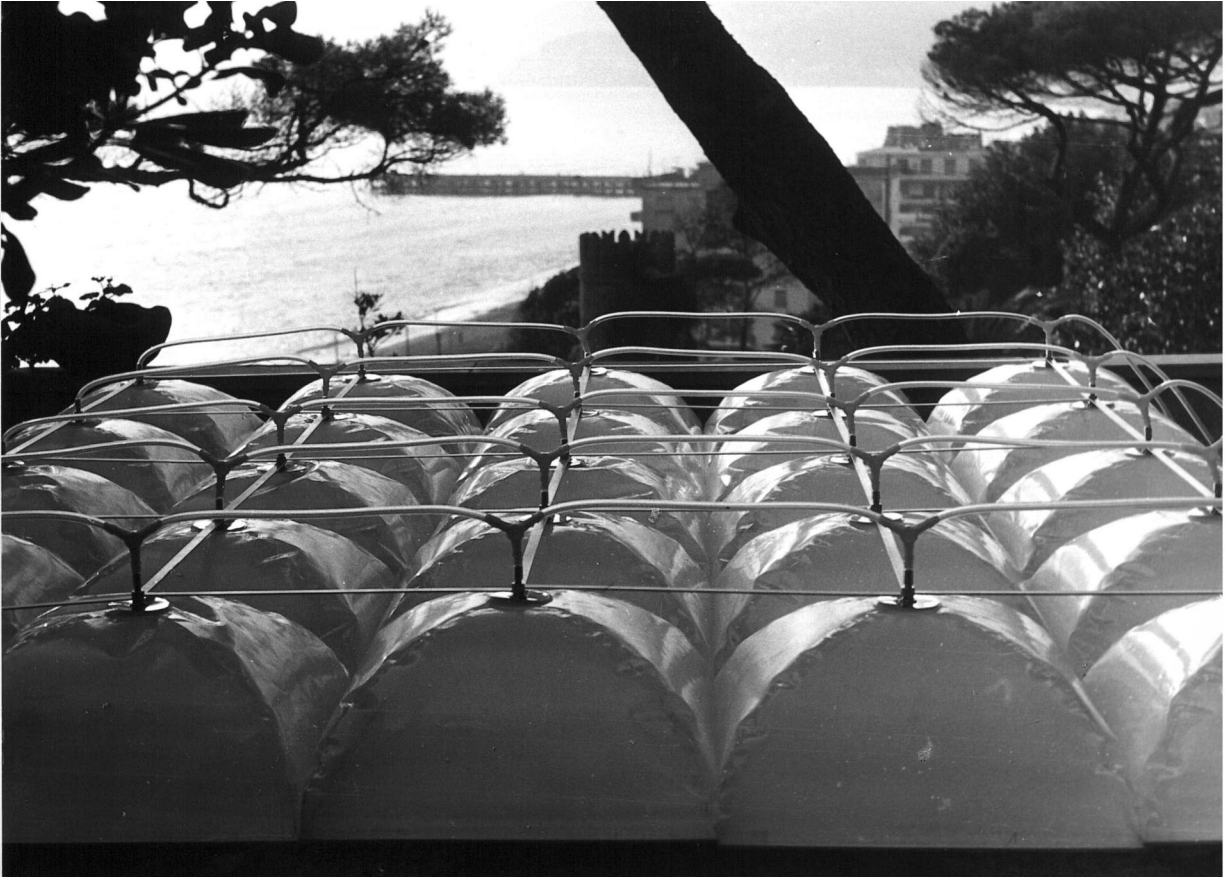
Figure 2: The structure in inflatable elements that Piano builds in the garden of his house in Genova Pegli in 1966.
