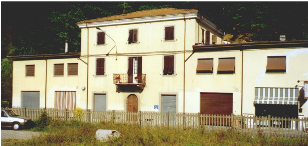
Figure 2. View of the building
