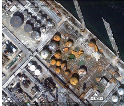
Figure 1.1: The LPG tank farm at the Chiba refinery after the earthquake-triggered fires and explosions.
