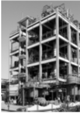
(a) Building like structures.
