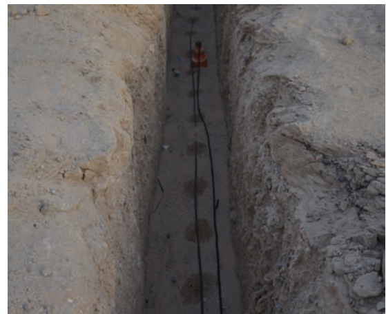
Figure 3 Installation and testing of the moisturizing network
