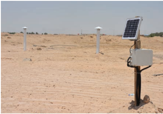
Figure 4 Installation of the data recording devices
