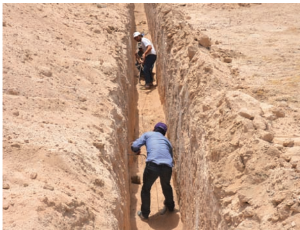
Figure 2 Preparation of the slope for the pipes
