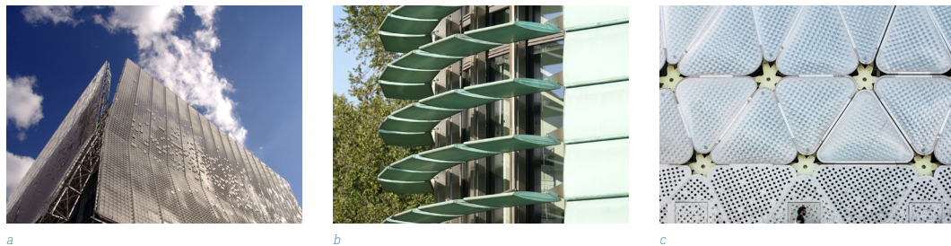
FIG. 1 Some pictures of active façades: a) ARTICULATED CLOUD, Pittsburgh (USA), 2004; b) Nordic Embassies in Berlin, Berlin (DE), 1999; c) MEDIA-TIC, Barcelona (SP), 2007
