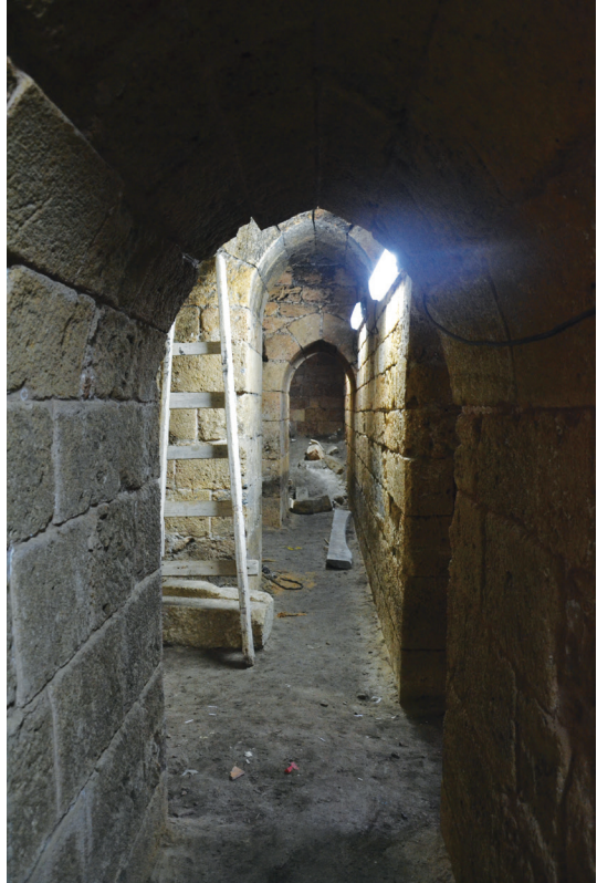
Fig. 8. The corridor of the hypogeum of the Sant'Andrea of Akko, which seems to populate the same foundation system designed to support a higher construction, today partly elided (author's photo)
