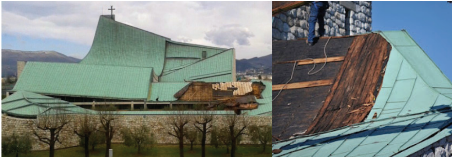
Figure 1. The San Giovanni Battista Church realized by Michelucci: the damage of the gallery of Nation roof after the storm
