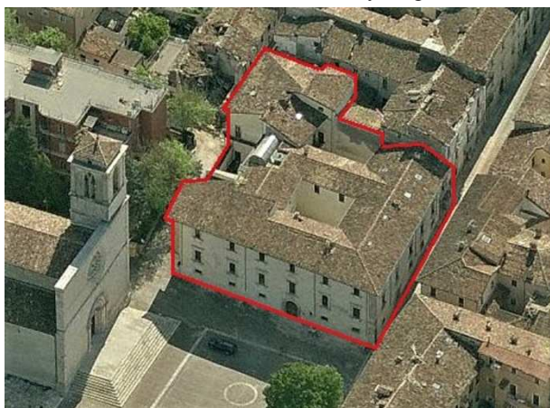
Figure 4. Palazzo Branconio, L'Aquila, Italy (picture taken from the author)
