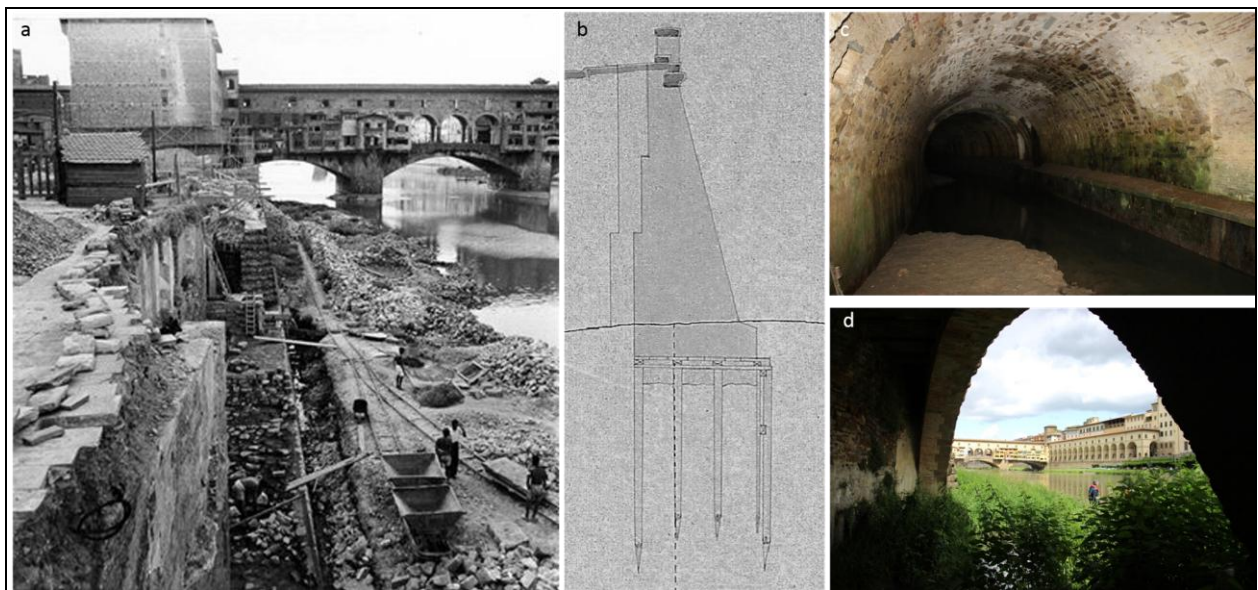
Figure 36. a) Original photo of the Torrigiani riverbank embankment at the beginning of its construction in 1866, (b) the section of the retaining wall from the original design drawings, and the discharge channel inside the Lungarno Torrigiani embankment, as visible in 2017 (c, d). (Morelli et al., 2018).
