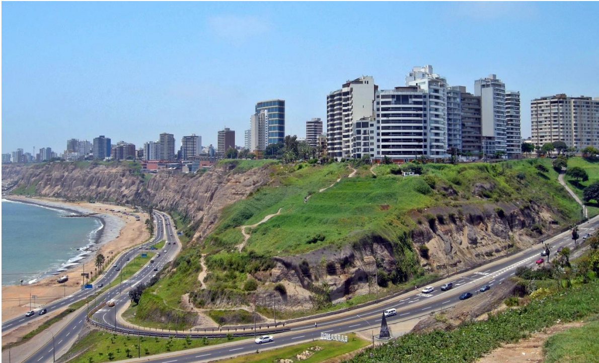
Photograph 2: Landslides control system, Miraflores neighbourhood, Lima, Peru.
