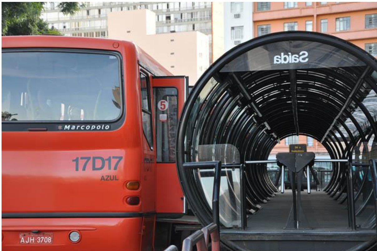
Photograph 8: A typical tubo station in Curitiba
