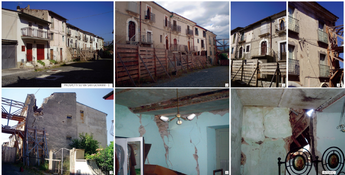
Figure 6-33: Castelnovo aggregate: façades and internal rooms.
