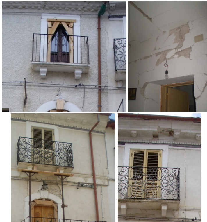
Figure 6-39: Castelnuovo aggregate: damage in the spandrels in S.U.6 (upper row) and in S.U.7 (bottom row).
