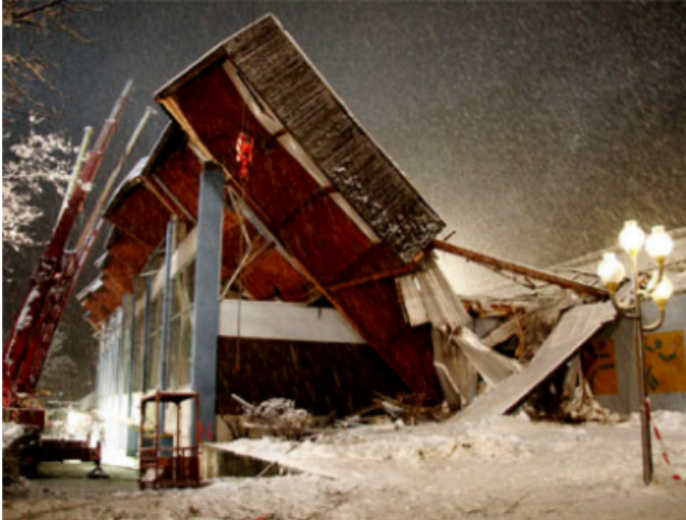
Figure 6.2: Roof collapse ice rink Bad Reichenhall [52].
