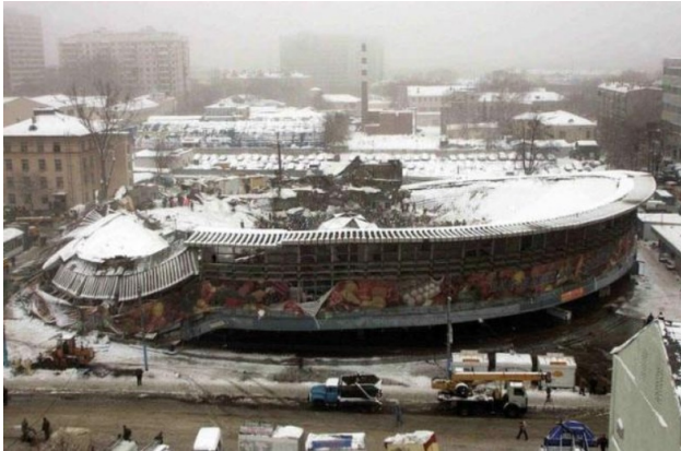
Figure 6.4: Roof collapse Basmanny Marketplace in Moscow.
