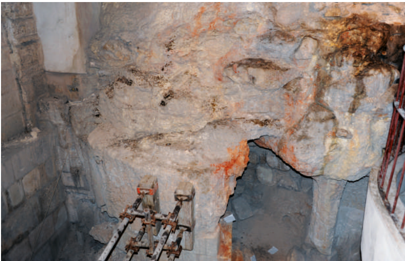
FIGURES 31 AND 32 Golgotha. On the 'point cloud' it is possible to observe the different masonry textures and therefore also distinguish the various construction phases of the building, starting from the bed rock up to the most recent works.
