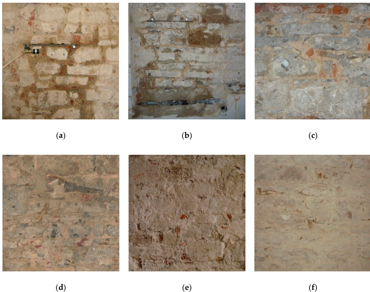
Figure 16. Masonry type III-1, ordinary public buildings—ID panels: (a) 064; (b) 075; (c) 076; (d) 077; (e) 090; (f) 092.
