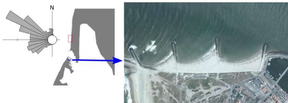
Figure 2-26 Example of a Groins field where the shoreline in the left side is turned against the prevailing wave direction; the latter can be deduced from the rose diagram on the right side of the image (Kristensen et al., 2016).
