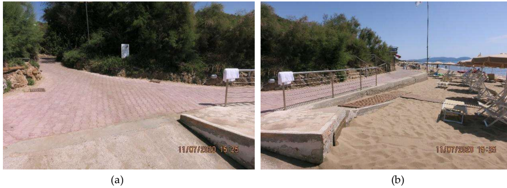
Figure 5-55. Artificial gangway from the touristic village to the shore at sectors 147, 148 and 149.
