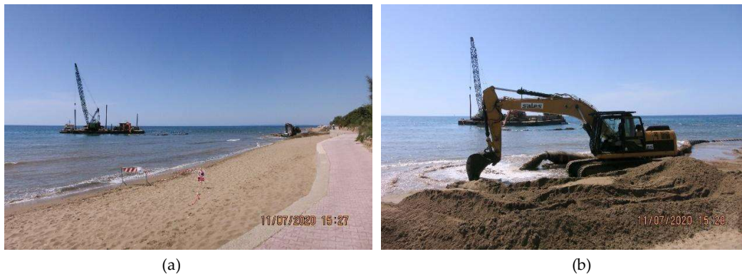
Figure 5-54. Artificial nourishment at sector 148.
