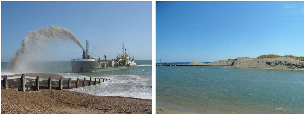
Figure 2-40 (A) Dredge during a beach replenishment in UK, image source: www.escp.org.uk/beach-nourishment ; (B) Dredged material at the harbor mouth at Laghi di Sibari, Crati river's mouth (Calabria, South of Italy).
