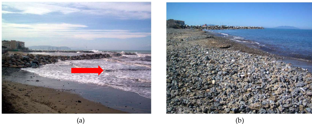
Figure 6-1 North harbor area (sector 134). (a) The red arrow shows the reflected wave by the breakwater during the working phase in 2006; (b) beach rock fragments used to nourish the erosive spot (Bianco et al., 2020).
