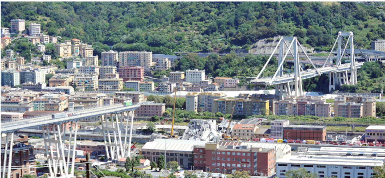
Figure 1-1 The partial collapse of Polcevera viaduct in the 14 th of August 2018, killing 43 people ( source ilpost.it ). The viaduct also known as the Morandi bridge from the name of its designer, the Italian engineer Riccardo Morandi, was built in the 1967 with a system of prestressed cable system innovative for that period. The bridge suffered degradation problems due to the corrosion of the steel cables and rebars.
