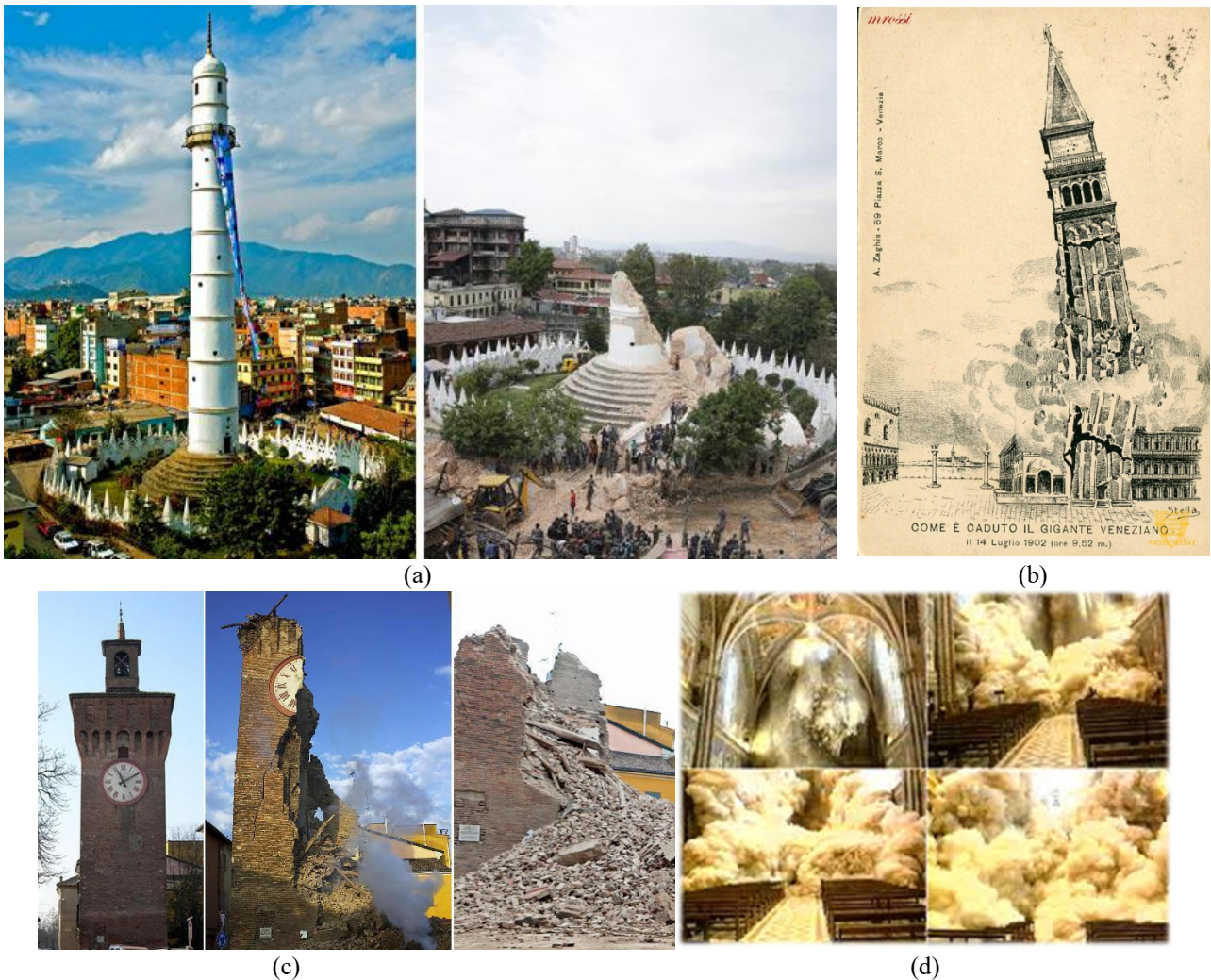
Figure 1-II (a) The Dharahara tower in Katmandu before and after the magnitude 7.8 earthquake in Nepal in April 2015 ( source nextquotidiano.it ). (b) the collapse of the San Marco bell tower in Venice in July 1902 (illustrated postcard, source venipedia.it ). (c) The collapse of the clock tower in Finale Emilia after the Emilia Romagna earthquake in the 2012. (d) The sequence of the vault collapse in the San Francesco's church in Assisi during the 1997 earthquake.
