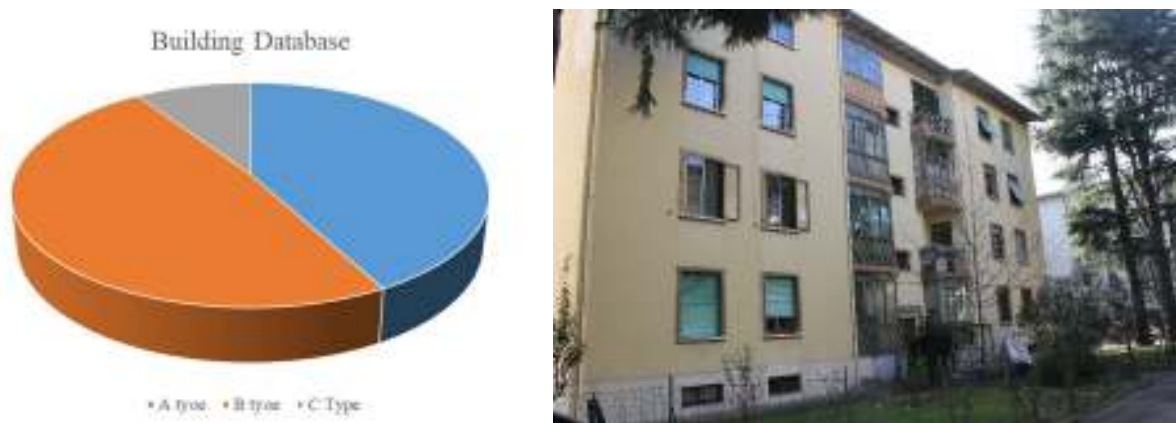
Figure 2.6. On the left: classification of the database from the relationship of the building levels with the soil. On the right: an example of public house with underground cellars.
