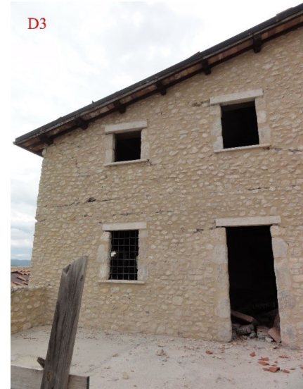
Figure 4.15: Damage Class “D3” assigned to the SU 114 according to the Gregorian Cadastre.
