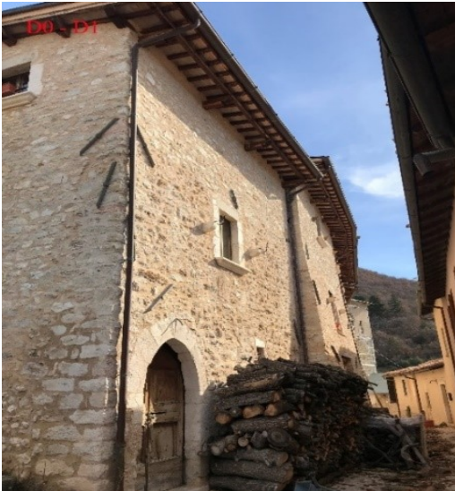
Figure 4.13: Damage Class "D0-D1" assigned to the SU 197 according to the Gregorian Cadastre.
