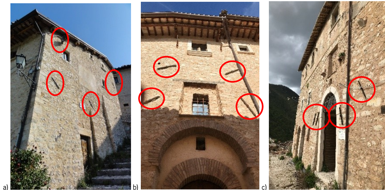
Figure 6.18: The number and distribution of metal ties, highlighted in red, leads to the assignment of class A (a), B (b) and C (c) for the buildings identified.
