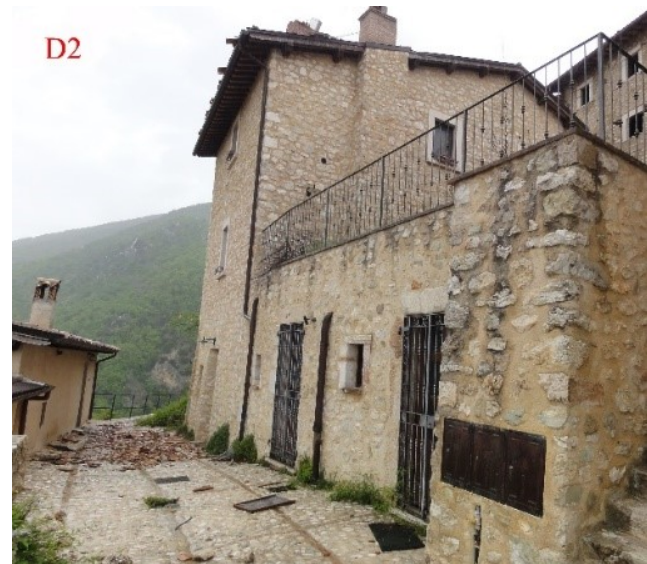
Figure 4.14: Damage Class "D2" assigned to the SU 1019 according to the Gregorian Cadastre.
