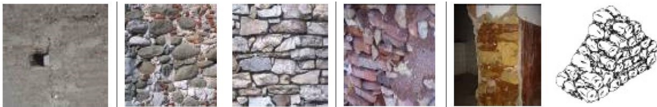
Figure C. 4: Masonry typologies identified for class D.
