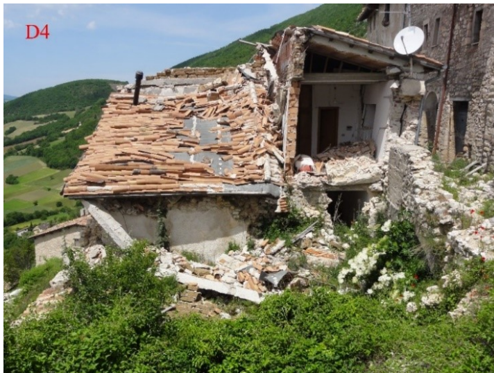
Figure 4.16: Damage Class “D4” assigned to the SU 165 according to the Gregorian Cadastre.
