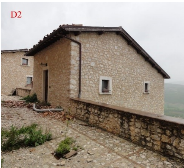
Figure 4.14: Damage Class "D2" assigned to the SU 1019 according to the Gregorian Cadastre.
