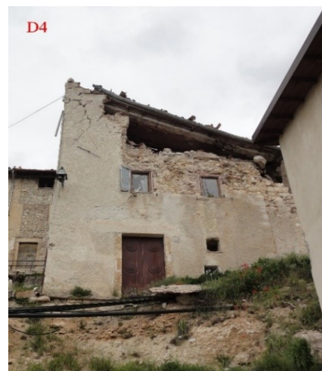
Figure 4.16: Damage Class “D4” assigned to the SU 165 according to the Gregorian Cadastre.
