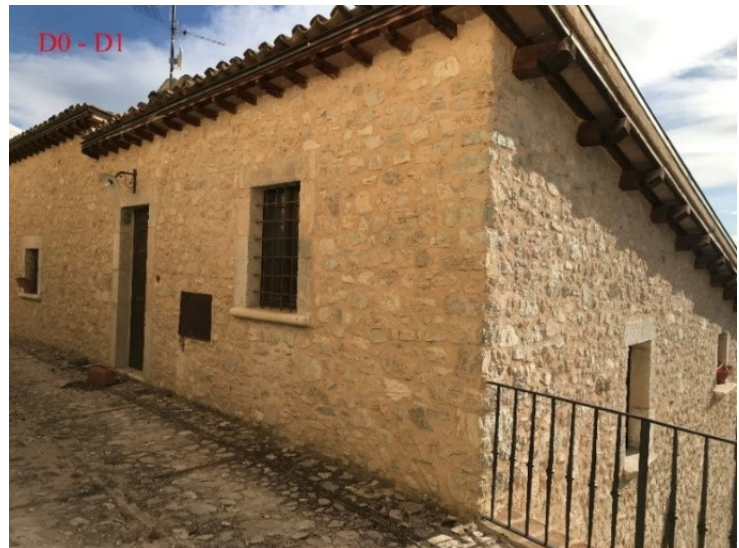
Figure 4.13: Damage Class "D0-D1" assigned to the SU 197 according to the Gregorian Cadastre.
