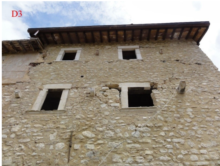
Figure 4.15: Damage Class “D3” assigned to the SU 114 according to the Gregorian Cadastre.
