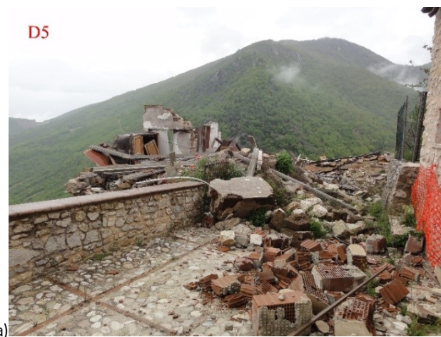
Figure 4.17: Damage Class “D5” assigned to the SU 54 according to the Gregorian Cadastre (a) and SU 54 before the earthquake (b).
