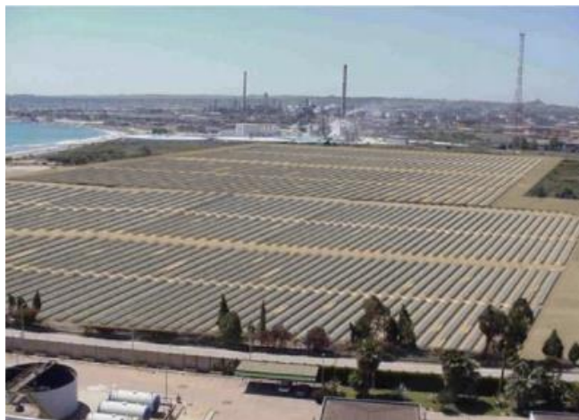
Figure 10. Archimede solar plant in Sicily [37].
