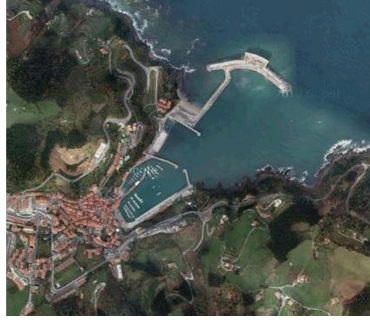
Figure 2.24: Image of the breakwater of the port of Mutriku embedding the multi-chamber OWC system [16].
