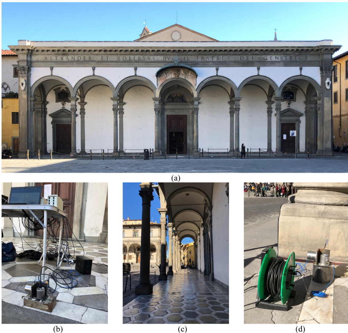
FIGURE 3 (a) Front view of the lodge from the SS. Annunziata's place (b) the DAQ system used during the test (c) lateral view inside the lodge (d) the triaxial measuring station made up with three piezoelectric accelerometers
