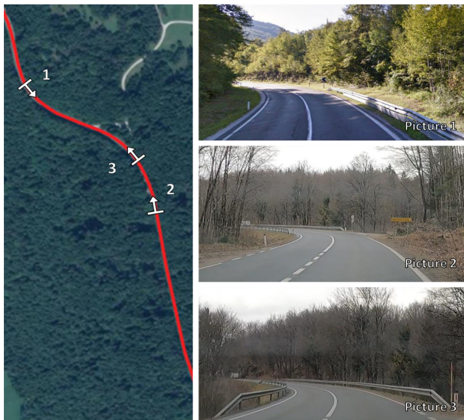
Appendix Figure 40 – NAS 9 of 106, view on satellite image and pictures of the road
