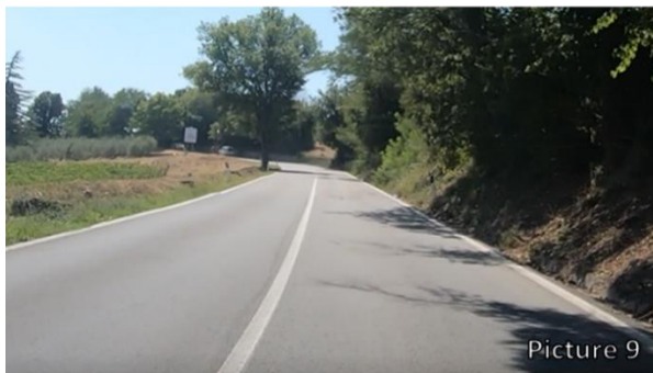
Appendix Figure 35 – Pictures from NAS 2 of SR2, southbound
