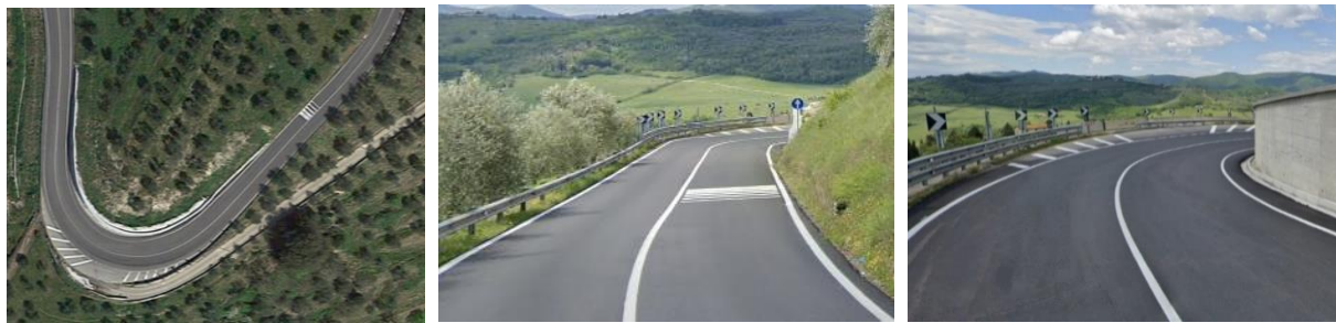
Figure 3.57 – Example of a critical curve, left - north oriented satellite view, right - photo approaching the curve from East. The curve is visible from distance but not understandable. The field of view shows many problems: the barrier line follows a different trajectory from the road axis, white markings along the shoulder create bad focus point and modify the perception of the road curvature (Andrea Paliotto, photos from Google Maps)
