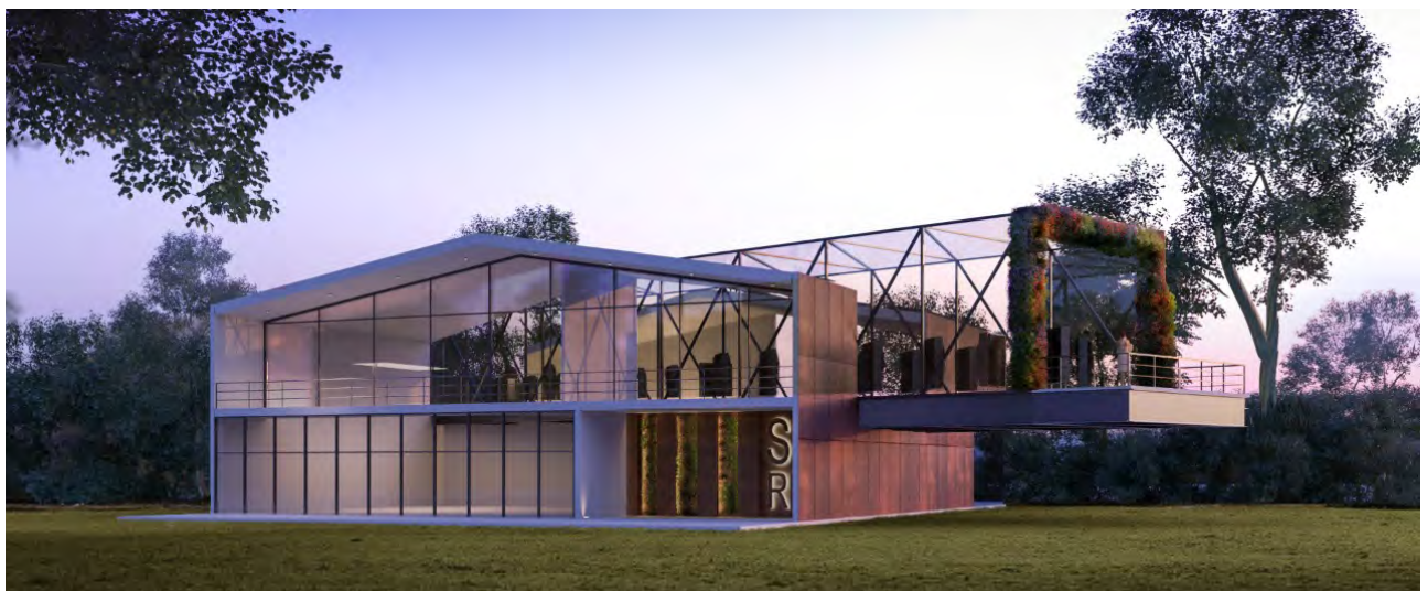
Main building exterior view 2
