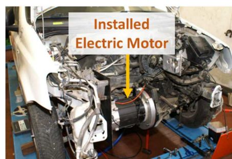
Fig. 4. Installatio of the electric motor in the Panda Prototype
