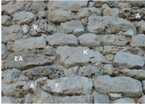
Fig. 5- Decay forms on the tower masonry. A= alveolation; EA= elongated alveolation (fissure); F= fracturing and flaking; K= karstification, (graphic elaboration by Fancello, 2022)
