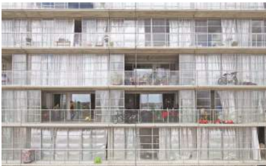
02. Facciata con pannellature scorrevoli prefabbricate di vetro | Facade with prefabricated sliding glass panels. Philippe Ruault
