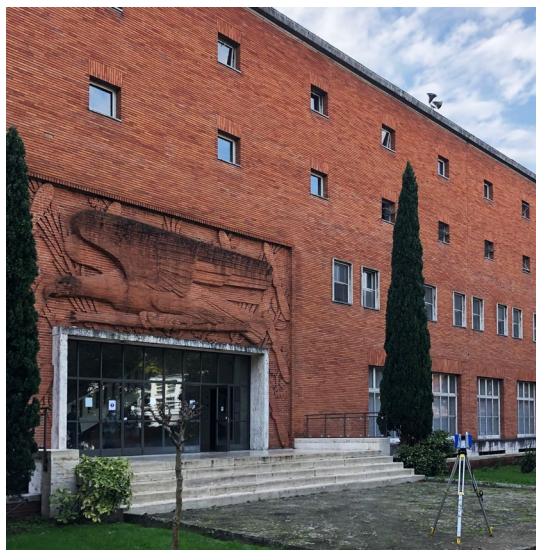
Fig. 9 - Range-based data acquisition phase using TLS
