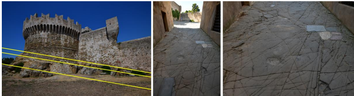
Fig. 2. The lines from the stone levels in the basement of the fortress and the stone cut to shape the floor of Populonia downtown.
