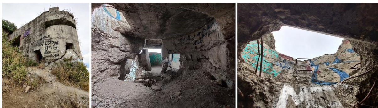
Fig.14. External and internal views of the bunkers in their present conditions.
