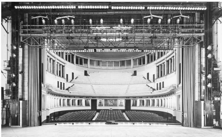
Fig. 2. Historical photograph taken from the stage, facing towards the audience, before 1940s works. Archivio Storico del Maggio Musicale Fiorentino.
