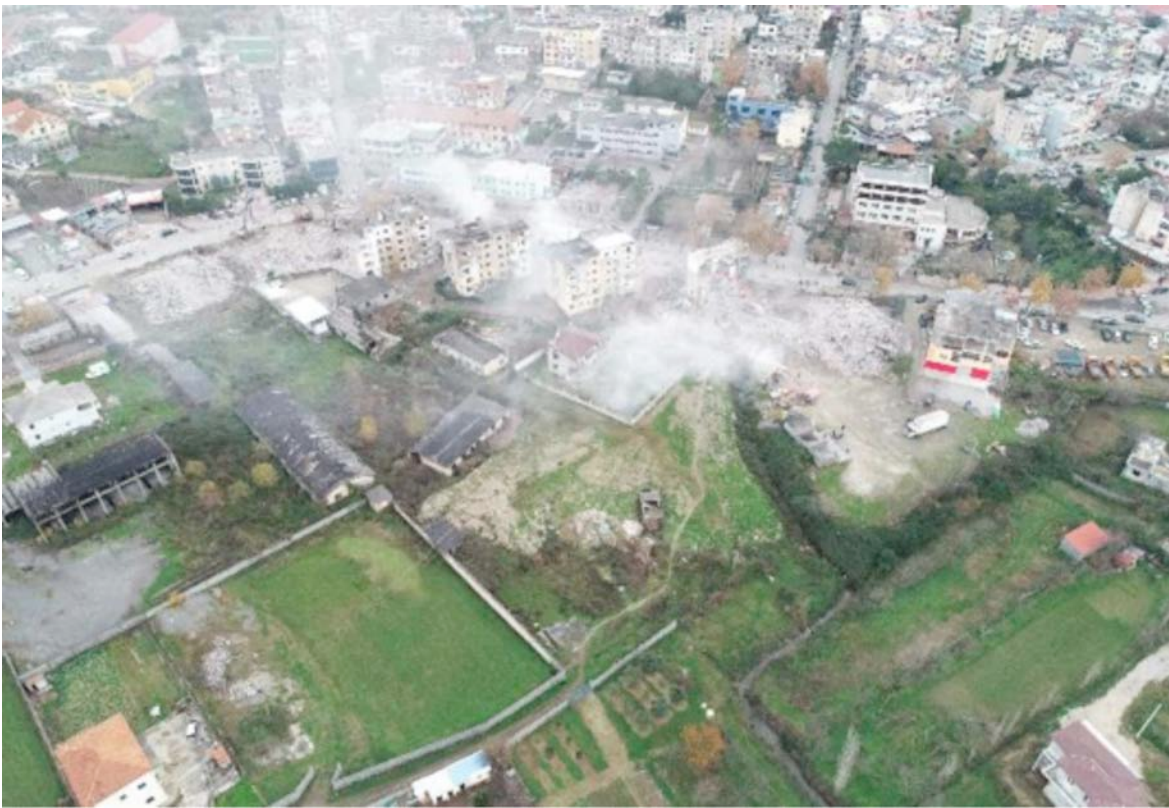
Fig. 1 Demolition of Damaged Buildings in New Development Area 1.1.
