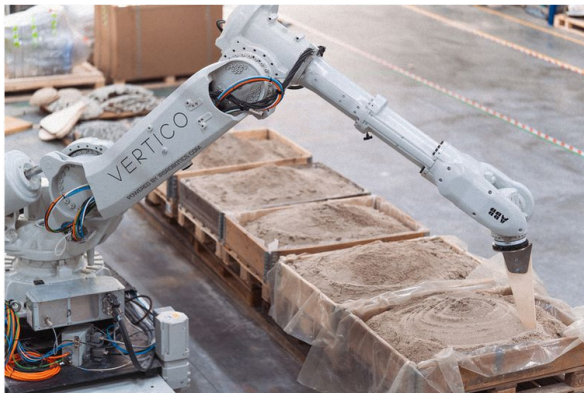
Figure 14. Case study 3D concrete printed facades (CS.09). Sand shape modelling is fully mechanised using multi-axis VERTICO robots (Source: VERTICO, [55]).
