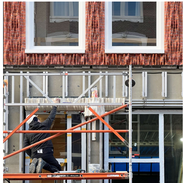
Figure 10. Case study Ceramic House (CS.01). Dry assembly of the ceramic finish (Studio RAP, photograph by Riccardo De Vecchi, [38]).
