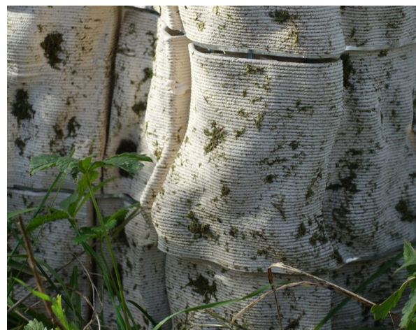
Figure 8. Case study Planter Tiles (CS.12). Prototype of the 3D-printed moss tiles fitted together to simulate a wall (Source: IOUS Studio, [66]).
