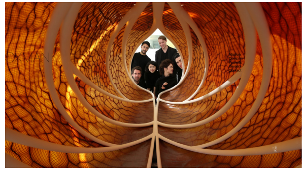
Figure 6. Case study Aguahoja I (CS.10). Interior view of the architectural pavilion made of biological compounds (including cellulose, chitin and pectin) of different densities (Source: OXMAN practice website, [62]).
