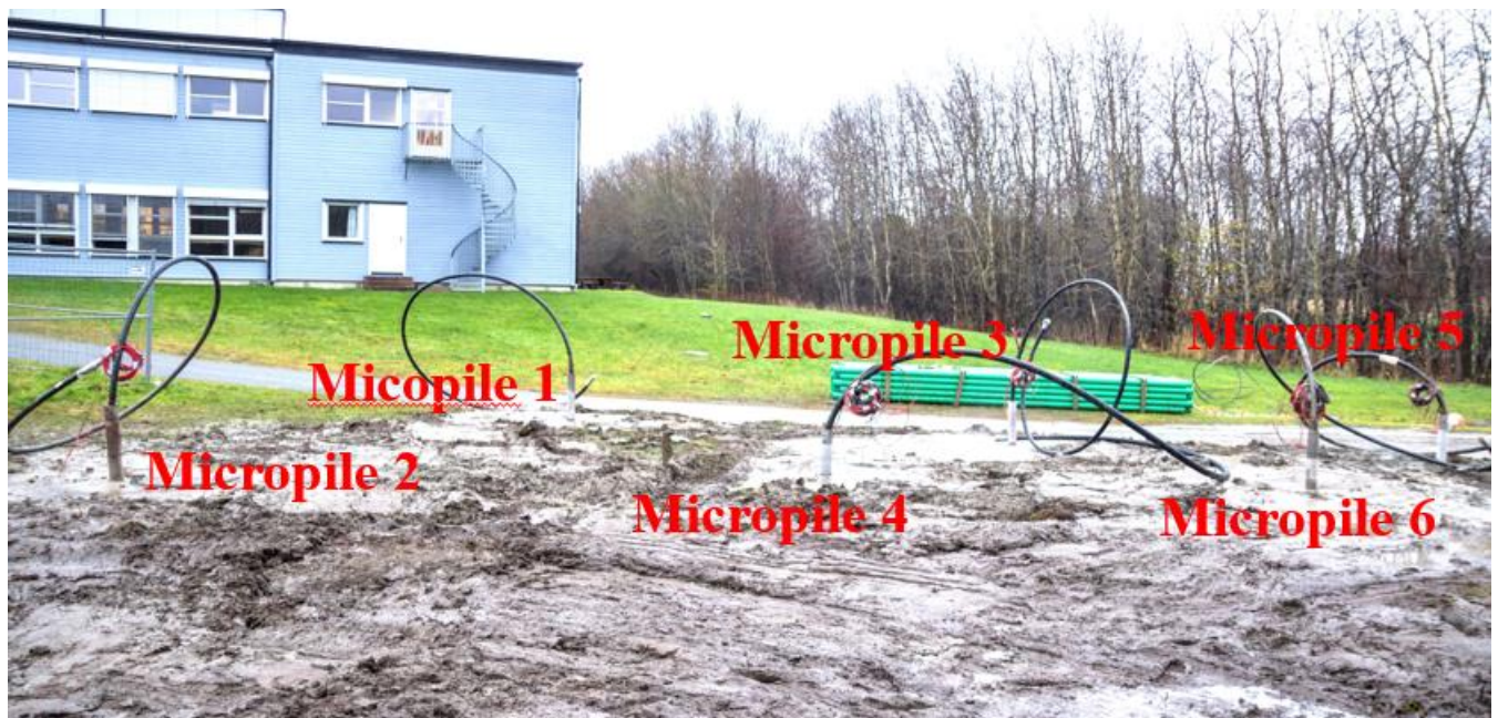
Figure 3.16: Installed micropiles on site (October 31, 2024).
