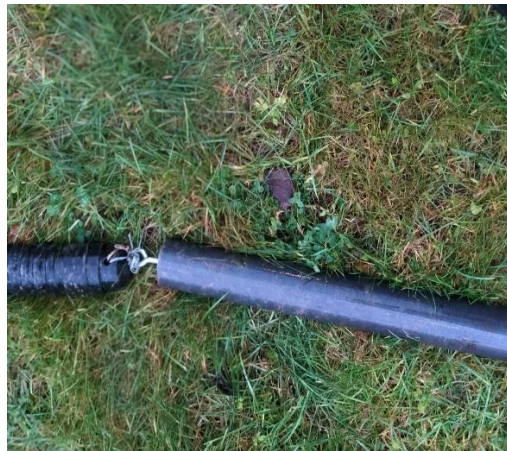
Figure 3.15: 10 kg load fixed to the bottom end of the coaxial pipe to ease pipe lowering in the hollow bar.
