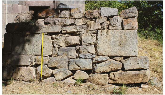
[fig. 5] B2 southern masonry with squared and smoothed re-used basalt ashlar and broken and roughly squared basalt blocks
