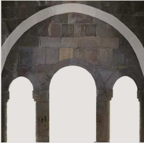
[fig. 8] The jutting relieving arch in ε5
