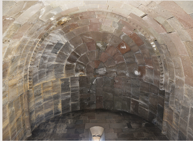
[fig. 9] The semi-dome and the barrel vault of the main apse in FUI
