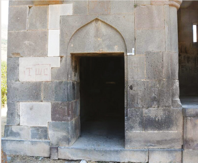
[fig. 10] Example of L-shaped notches and thinner ashlar used for the connection with the architectural elements (a segment of the right and left side of ε4)
