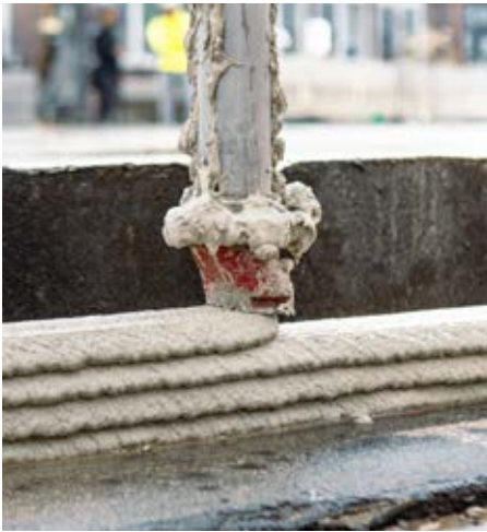
Fig. 4: Printing Process Wavehouse, ©SSV Architekten
