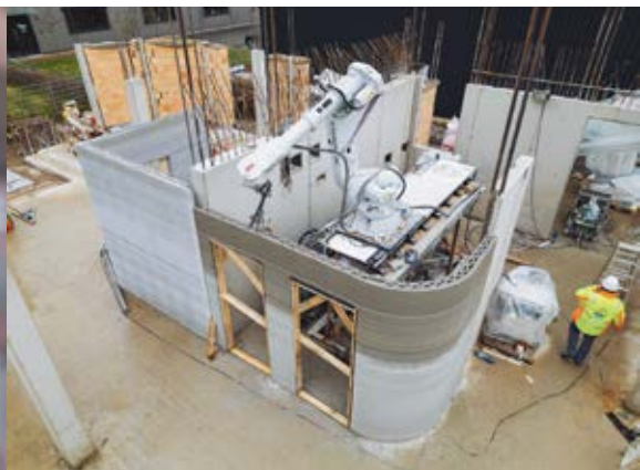
Fig. 3: Sirolis 3D Printing with Vertico technology ©Georgios
