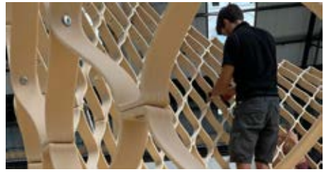
Fig. 4: Construction of the Biopolymer Pavilion
