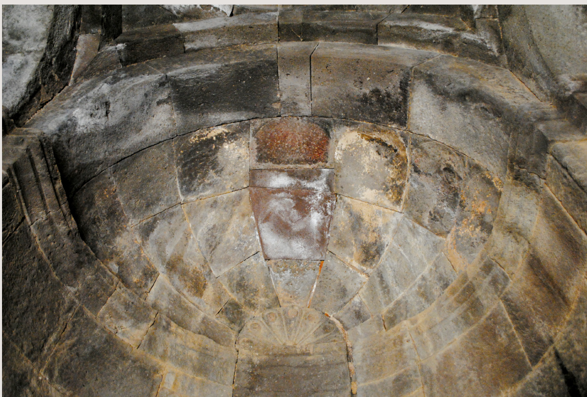
[fig. 6] The supporting system (double rounded arches and squinches) of the tambour and central dome
