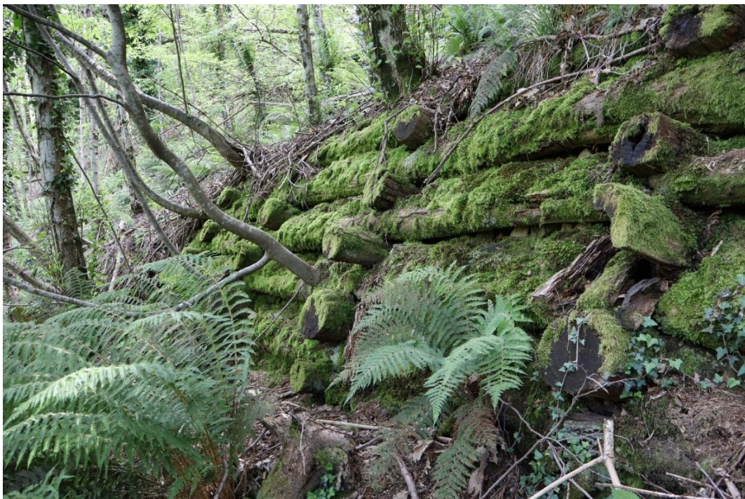
Figure 4: Live wooden crib wall during a 2023 field survey (pH. Emanuele Giachi)
