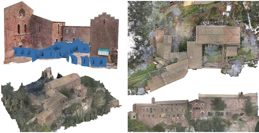
Figure 4.4: 3D photogrammetry close-range and by UAV of the Castell-Monestir de Sant Miquel d'Escornalbou, Tarragona, Spain.
