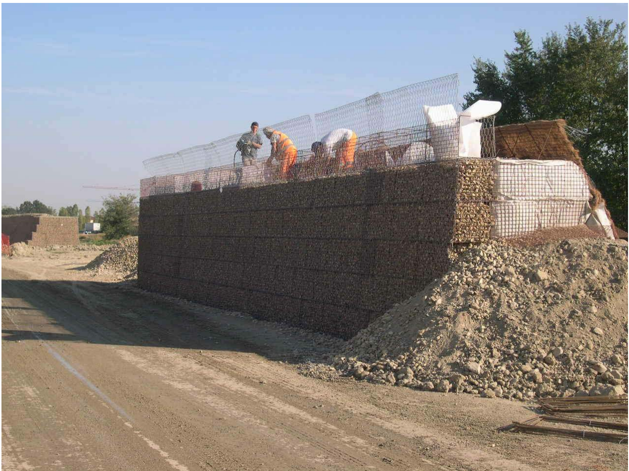
Figure 12 Photo showing the implementation of a test dune, with differentiated 60°/90° slopes, with vertical gabion faces
