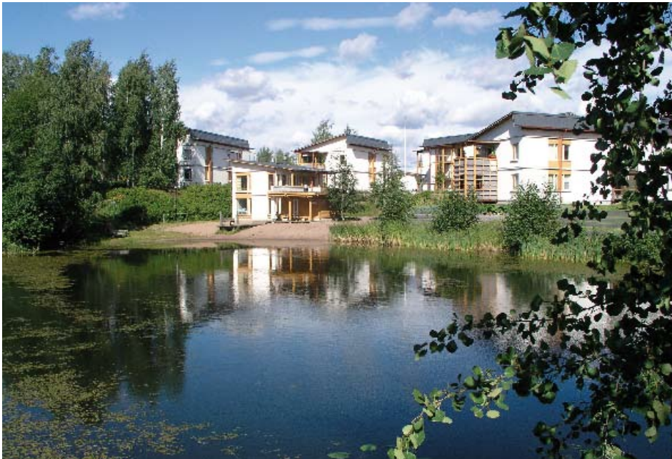
5. Experimental area for timber construction apartment buildings
