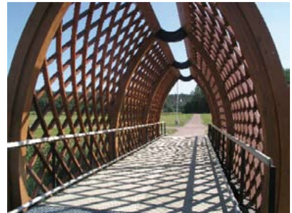
8. In Viikki's planning, green areas are considered to be an ecological perspective visible in the unbroken continuity of the overall open space entity. Pedestrian and cycle bridge over the Viikkinoja canal
